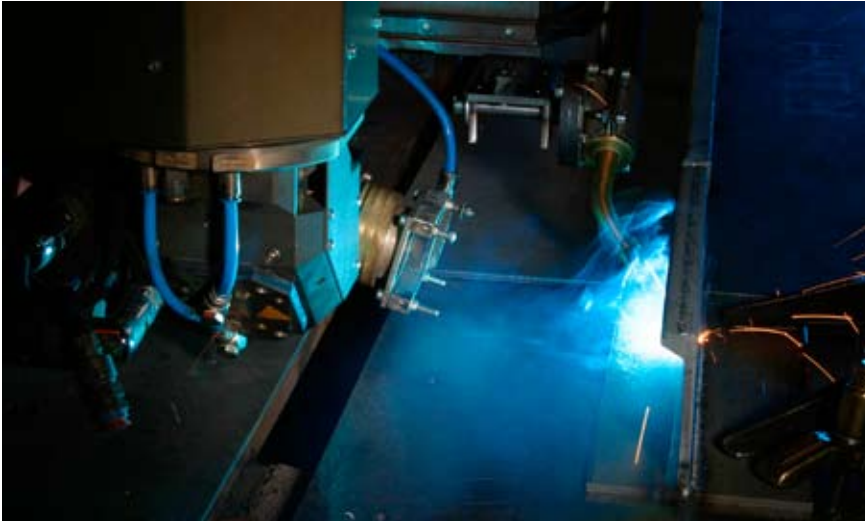
Fig. 6. Hybrid laser welding of a structural steel case.
